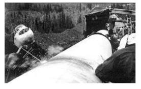
metal. Actual welding was controlled remotely. About 30 weld passes were required for each joint.
