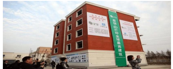
g. 31. 3D Printed Apartment Building by Winsun, 2015
